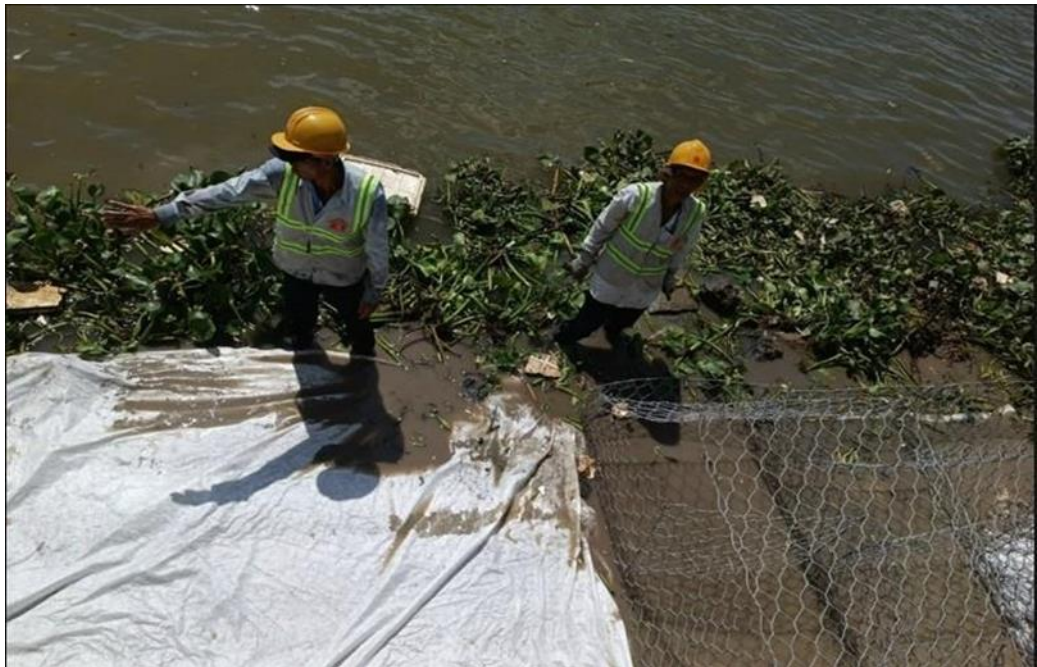
Using gabions + geotextiles in the project to prevent embankment erosion in Thu Duc City, HCM.
