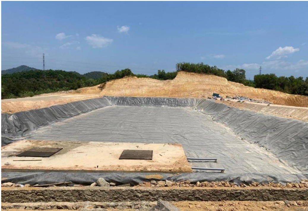
1.0mm HDPE geomembrane is used for landfill construction in Lam Dong province
