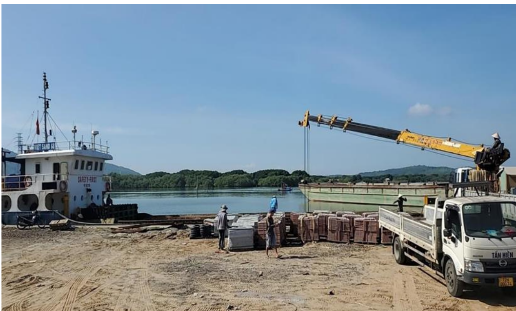
1.0mm HDPE geomembrane is used for freshwater reservoir construction in Con Dao, Ba Ria - Vung Tau province
